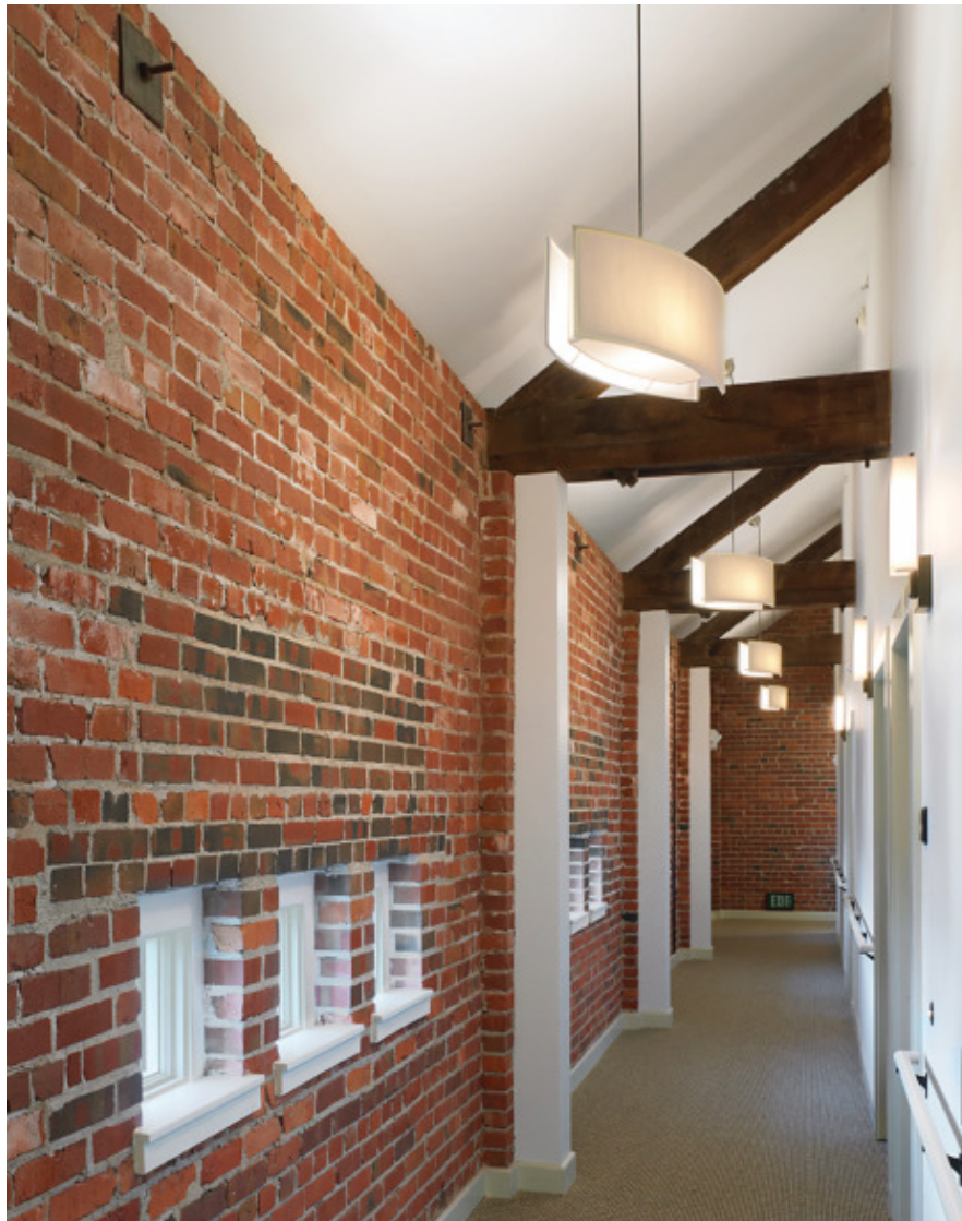
Image 9. Corridor with historic fabric columns. Source: Van Meter Williams Pollack archive
